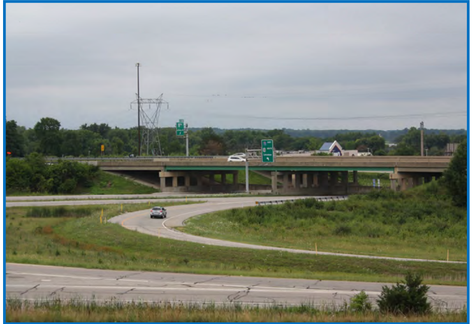
Photo 12—View of the I-70/US 40 Interchange Facing Southwest (07/26/2022).
