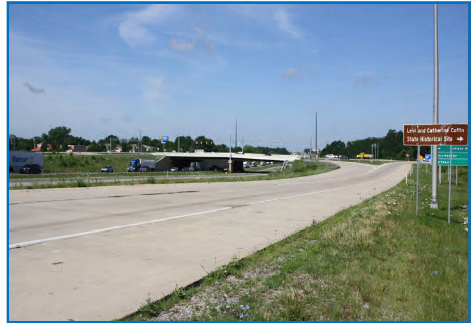
Photo 8— View of I-70 Approaching the US 27 Interchange Facing East (07/26/2022).
