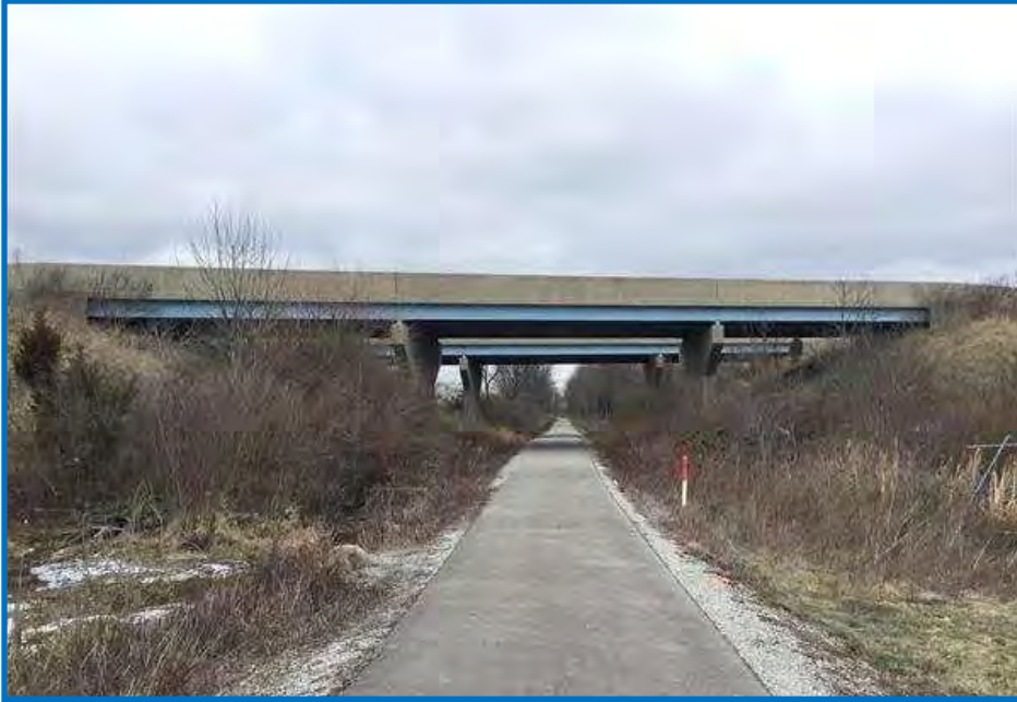
Photo 9— View of Cardinal Greenway Trail and EB and WB I-70 Bridges Facing South (01/21/2020).
