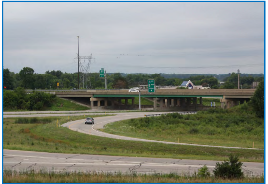
Photo 12—View of the I-70/US 40 Interchange Facing Southwest (07/26/2022).
