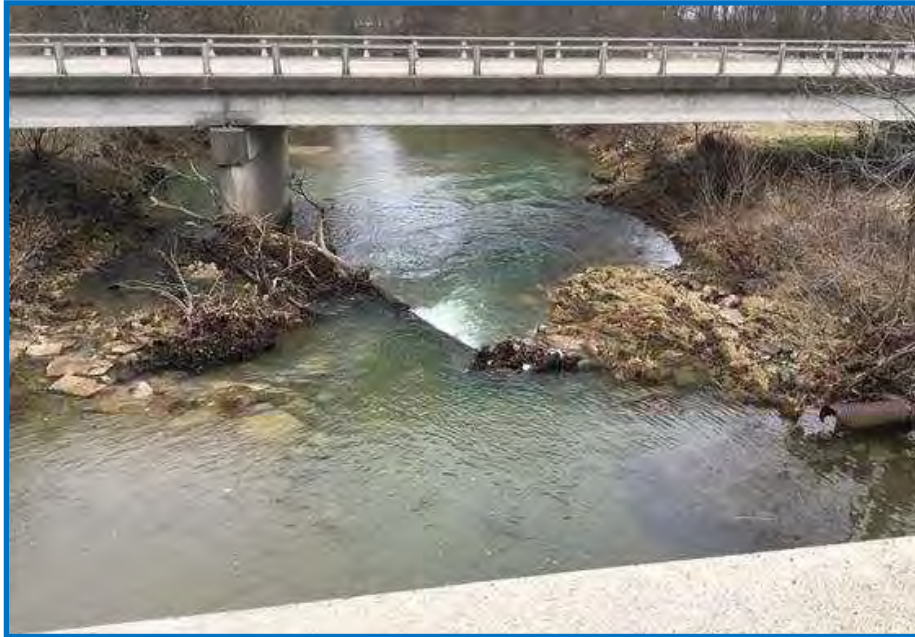
Photo 3 —View of Martindale Creek and the EB I-70 Bridge Facing North (01/28/2020).
