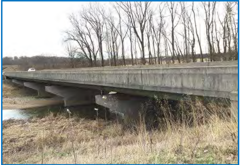
Photo 4 —View of the EB I-70 Bridge over Greens Fork (01/09/2020).
