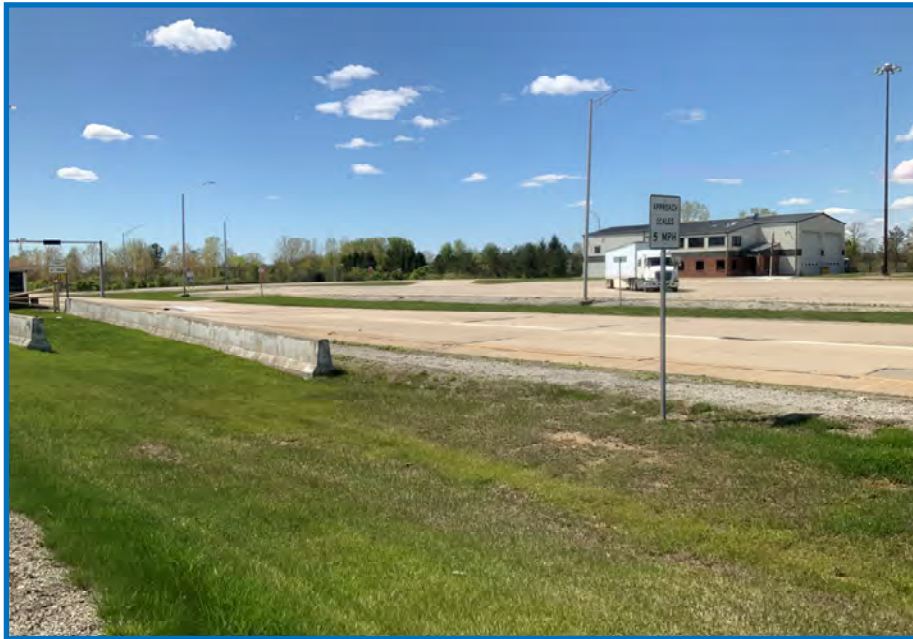
Photo 11- View of Weigh Station Facing West (05/05/2023)
