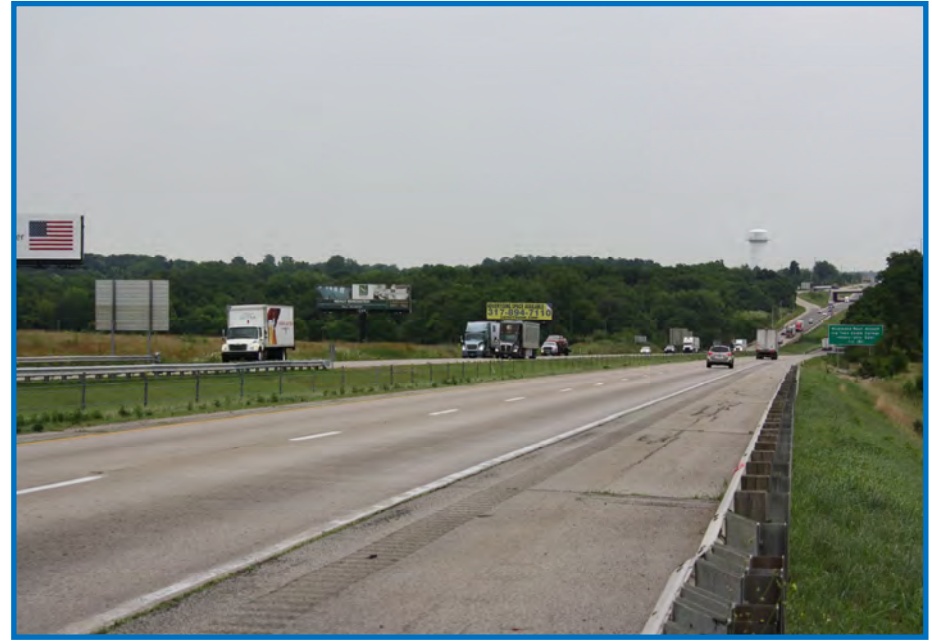
Photo 6—View of I-70 Approaching the US 27 I-70 Interchange Facing East (07/26/2022).
